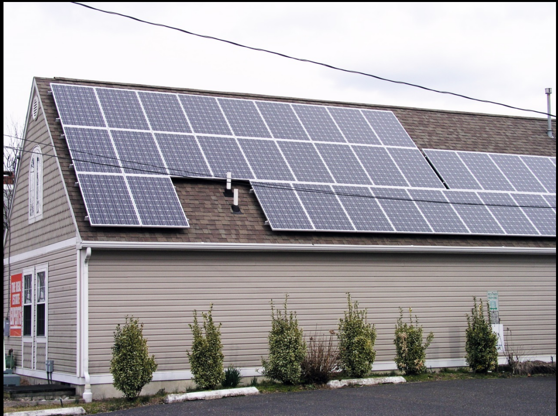
Above: Solar panels in Pemberton Township.
